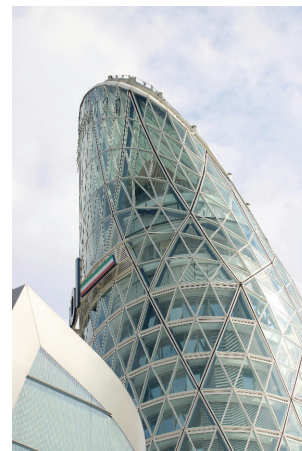
Figure 2.2. - High rise with a Diagrid Structural System located in Milano, Italia © Earth Photart, Pexels.com
