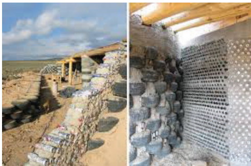
Figure 4.16. - Earthships (global) made of tire walls © nbcnews
