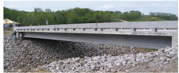
Figure 2.4. – You're looking at the first UHPC bridge constructed in the United States; Location: Wapello County, Iowa © FHWA DOT
