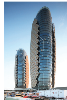
Figure 4.31. – Al Bahar Tower 1 in Abu Dhabi, United Arab Emirates © Aedas, Skyscrapercenter.com
