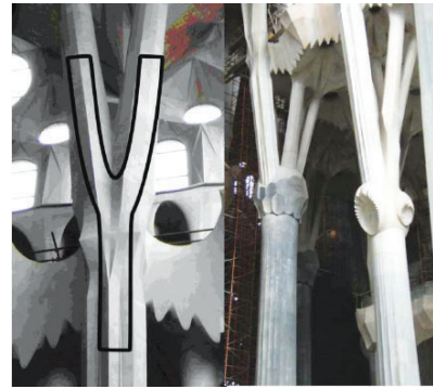
Figure 2.8. - The Columns of La Sagrada Família in Barcelona, Spain by Antoni Gaudí © Julian Francis Vincent, Research Gate
