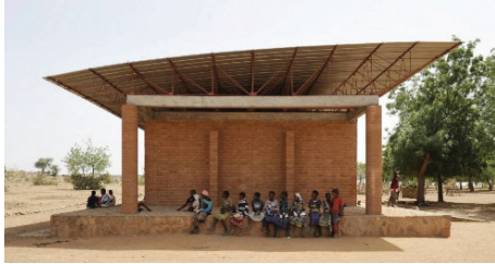
Figure 4.15. - Students sitting in the shade of Gando Primary School, Gando, Burkina Faso, Afrika © Erik-Jan Ouwerkerk, kerearchitecture.com
