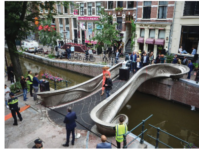
Figure 4.17. - MX3D 3D-printed steel bridge, Amsterdam (2021) © friedmanbenda.com
