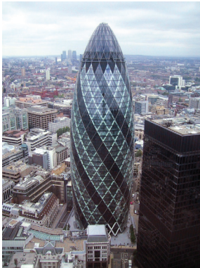
Figure 4.37. - The Gherki aka 30 St Mary Axe aka the Swiss Re Building © Wikipedia
