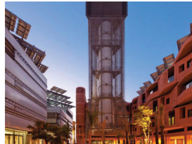
Figure 4.21. – Masdar City wind towers & solar chimney prototypes © solarchitecture.ch
