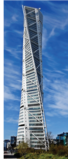
Figure 2.6. – HSB Turning Torso by Santiago Calatrava is based on Twisting Torso, a white marble sculpture by Calatrava; Location: Malmö, Sweden
