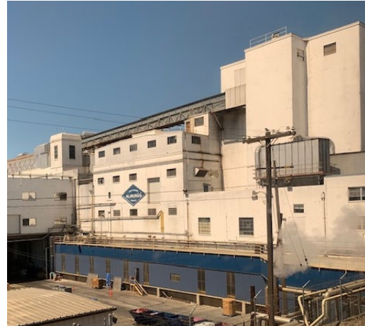
"Fit for Purpose" Industrial building – Western USA. Photo: Author 2021
