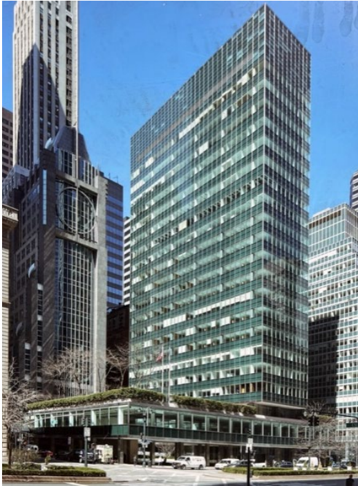
Original Lever House (SOM), New York, NY. 1952. Photo: Author 2022
