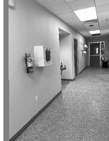
Protruding Objects – AED Cabinet and Fire Extinguisher
