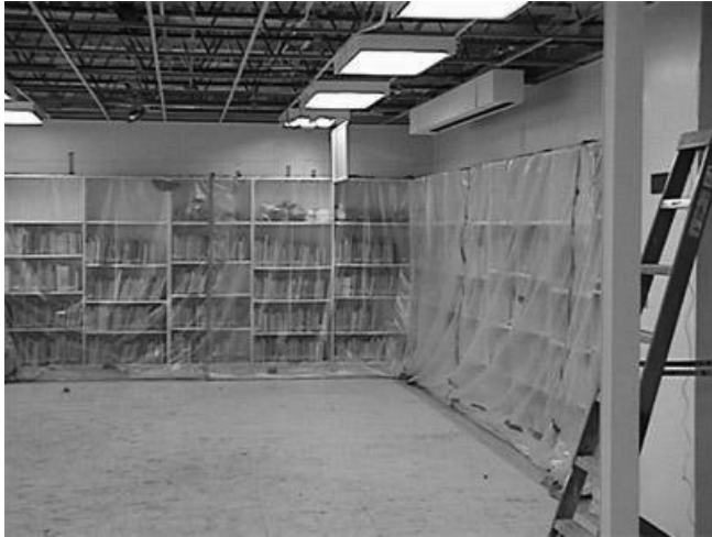
Minimizing further damage during restoration
