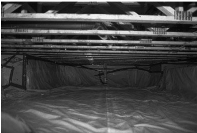
Properly protected crawl space
