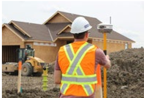
Surveying a construction site using a GPS receiver unit Source: United States Government
