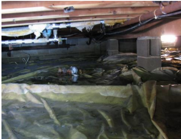
Flooded Crawlspace
