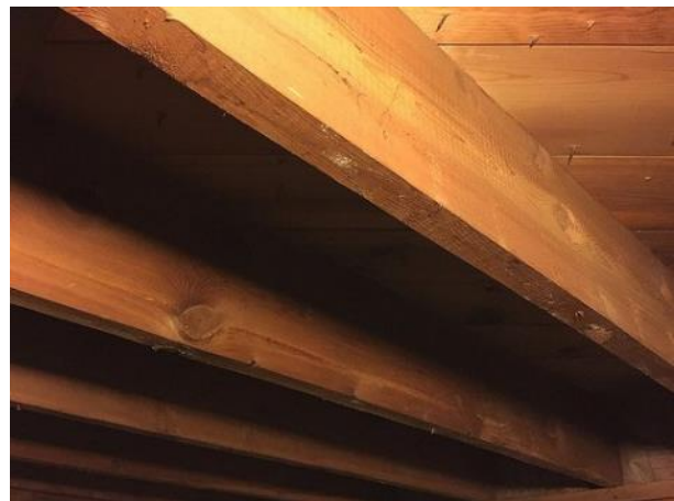
Floor Joist Framing
