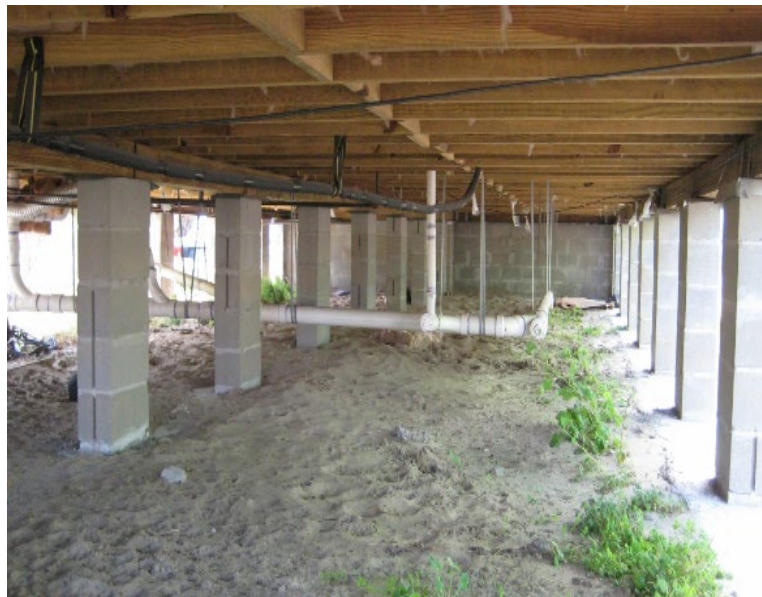
Open Crawl Space
