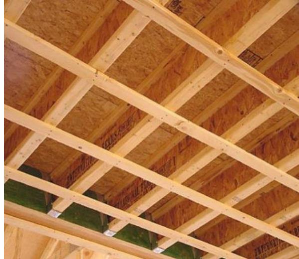
I-Joist Framing
