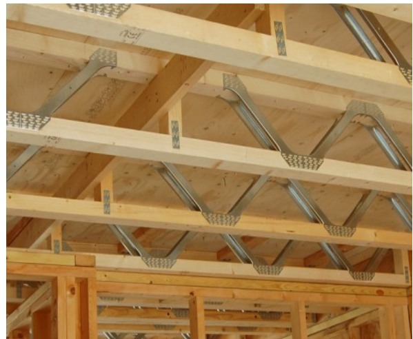
Floor Truss Framing
