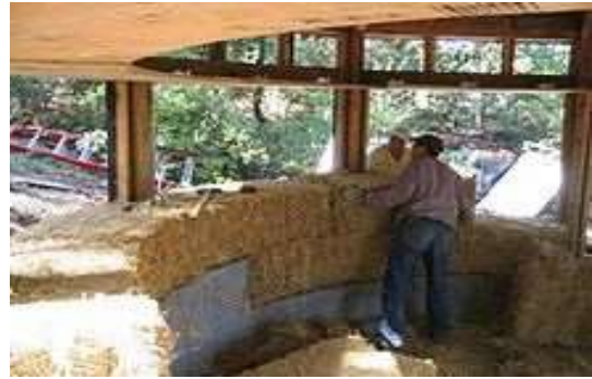
Building with Straw Bales
