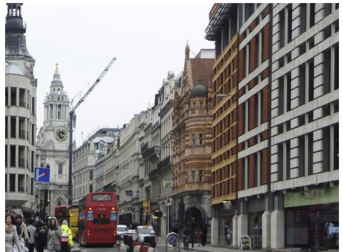
Figure 2.5. Mixed-use building, Ludgate Hill, London, 1999. Cullinan Studio, architects. Note how the articulation and materiality of the façade vary across its length to relate to the very different colors and materials in the adjacent buildings.
