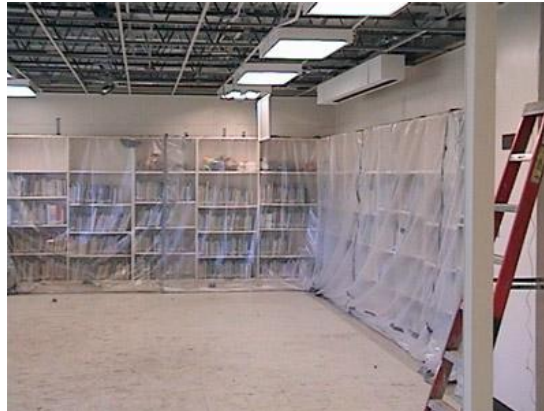
Minimizing further damage during restoration
