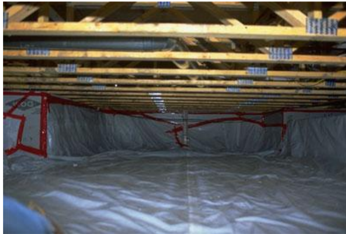
Properly protected crawl space
